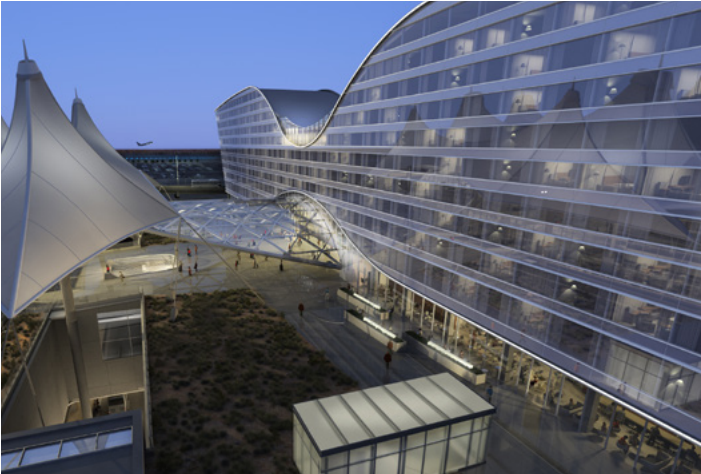
The South Terminal Redevelopment Program at Denver International Airport links it by transit to downtown Denver and creates a mixed-use destination at DIA anchored by a civic plaza.
