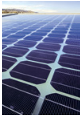
above: The design incorporates energy-producing photovoltaics into the building fabric.
