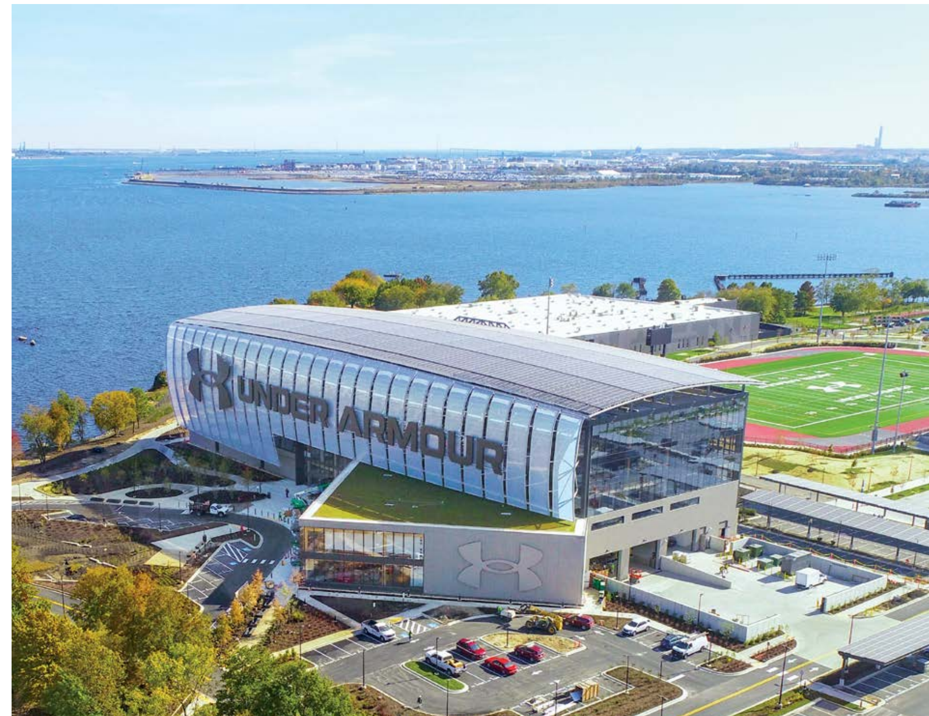
Under Armour Global Headquarters, Baltimore, MD This new mass-timber constructed HQ will pursue net zero energy operations along with WELL Building Standard and LEED v4 Platinum certifications.
