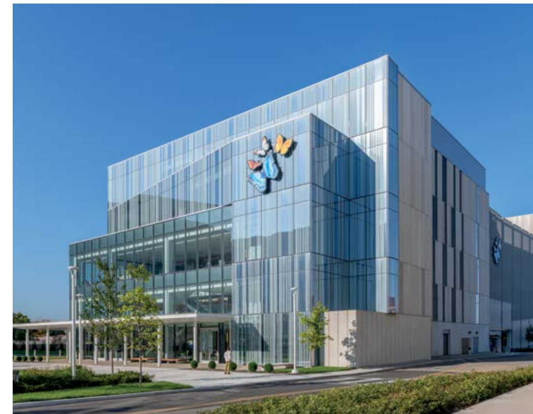
Nationwide Children's Hospital Data Center + Conference Facility, Columbus, OH
